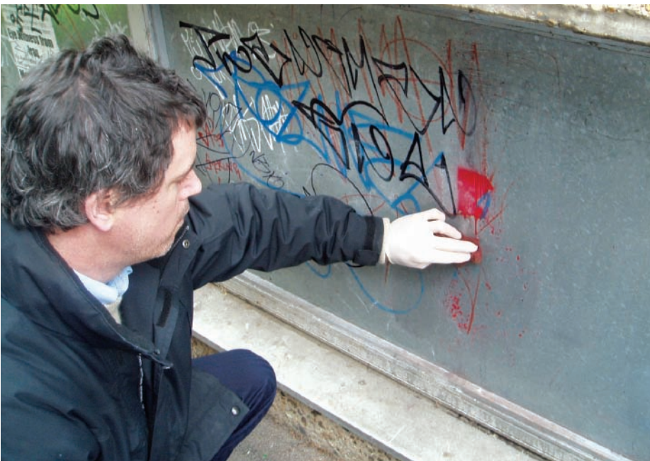
Removing graffiti using Graffiti Go™
