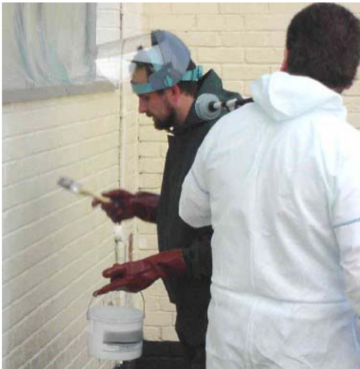
Photograph 1: Application of the paint stripper with a brush
