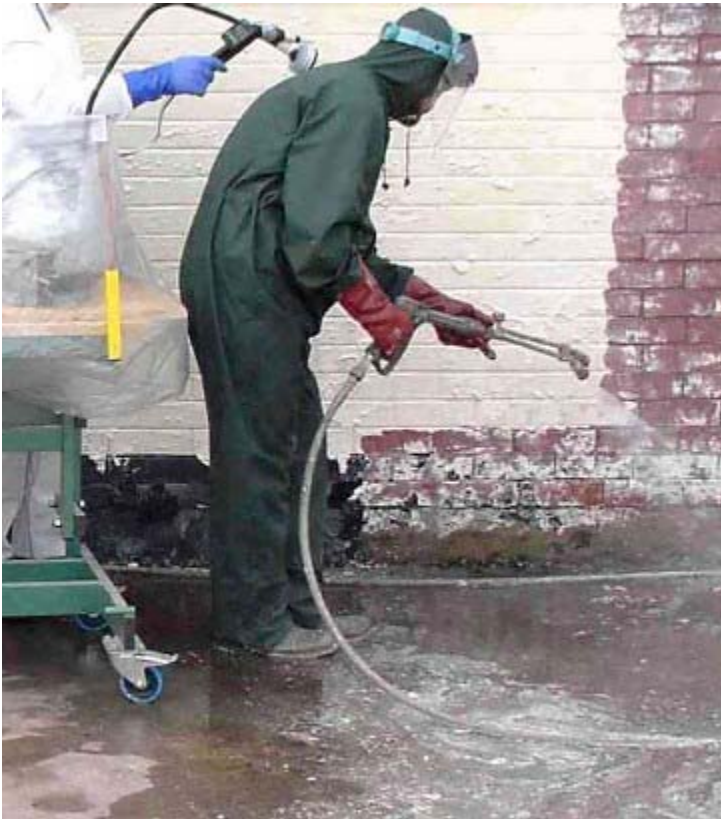
Photograph 2: Removal of the paint dissolved in the stripper with a hot water spray gun
